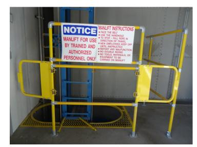
A certification record must be kept for each inspection to include the date of the inspection, signature of the person who performed the inspection, and the serial number or other identifier of the manlift which was inspected.
